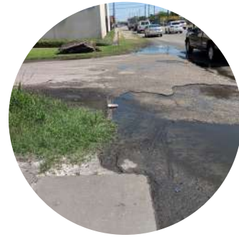
Fig 16: Roadway Ponding
