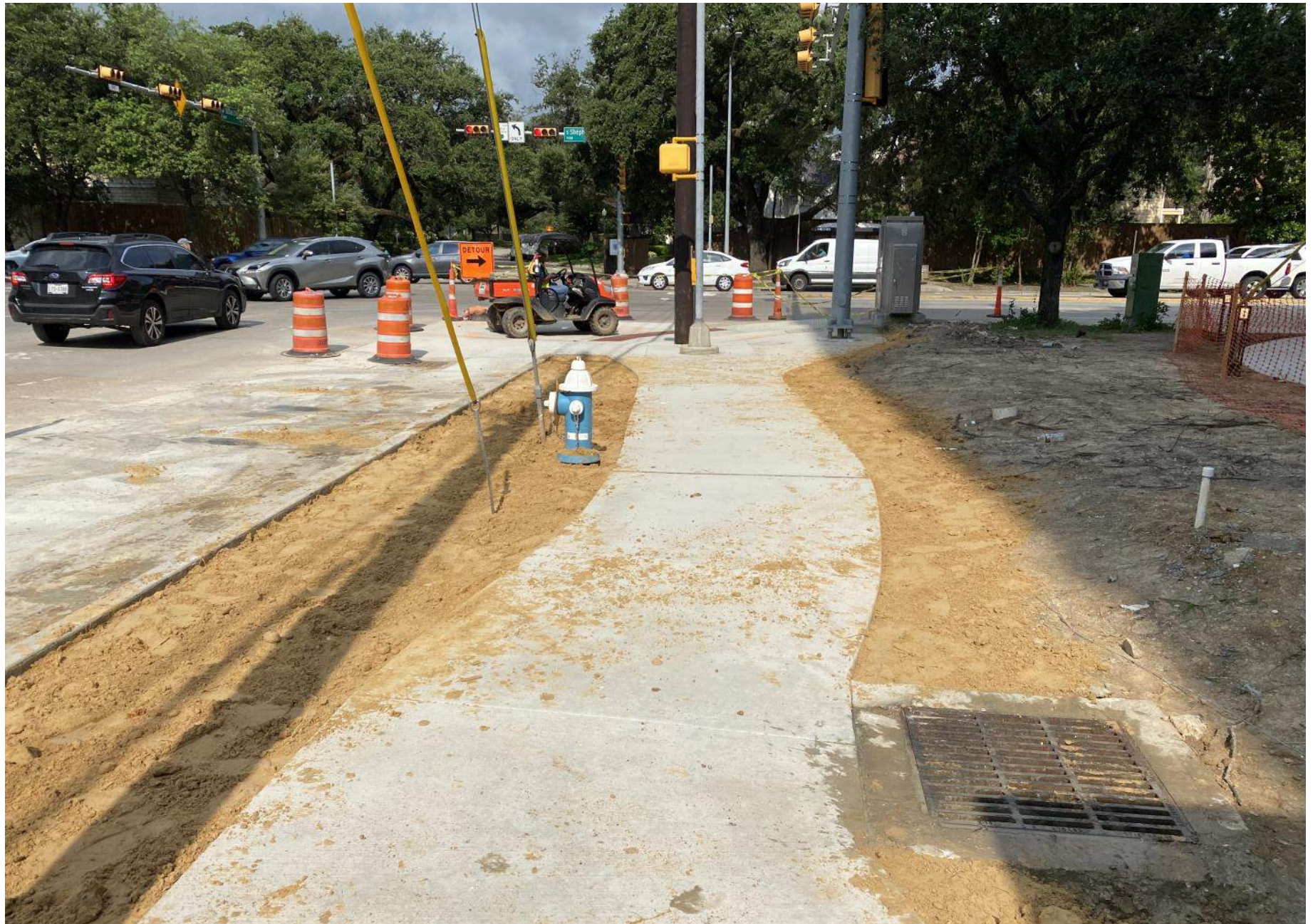
Fine grading on W. Dallas after paving and sidewalks
