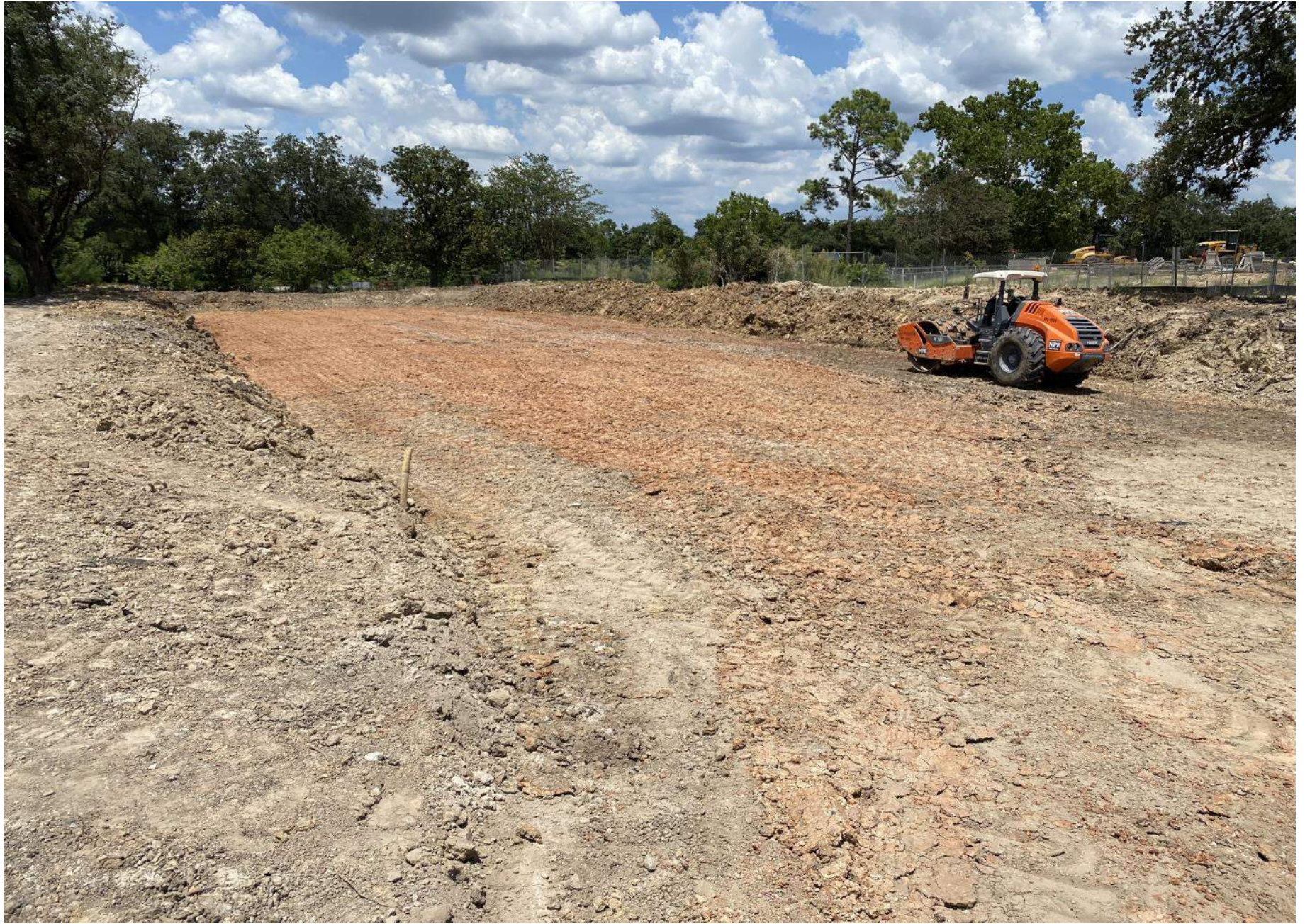
Continued backfill & grading at site “C”
