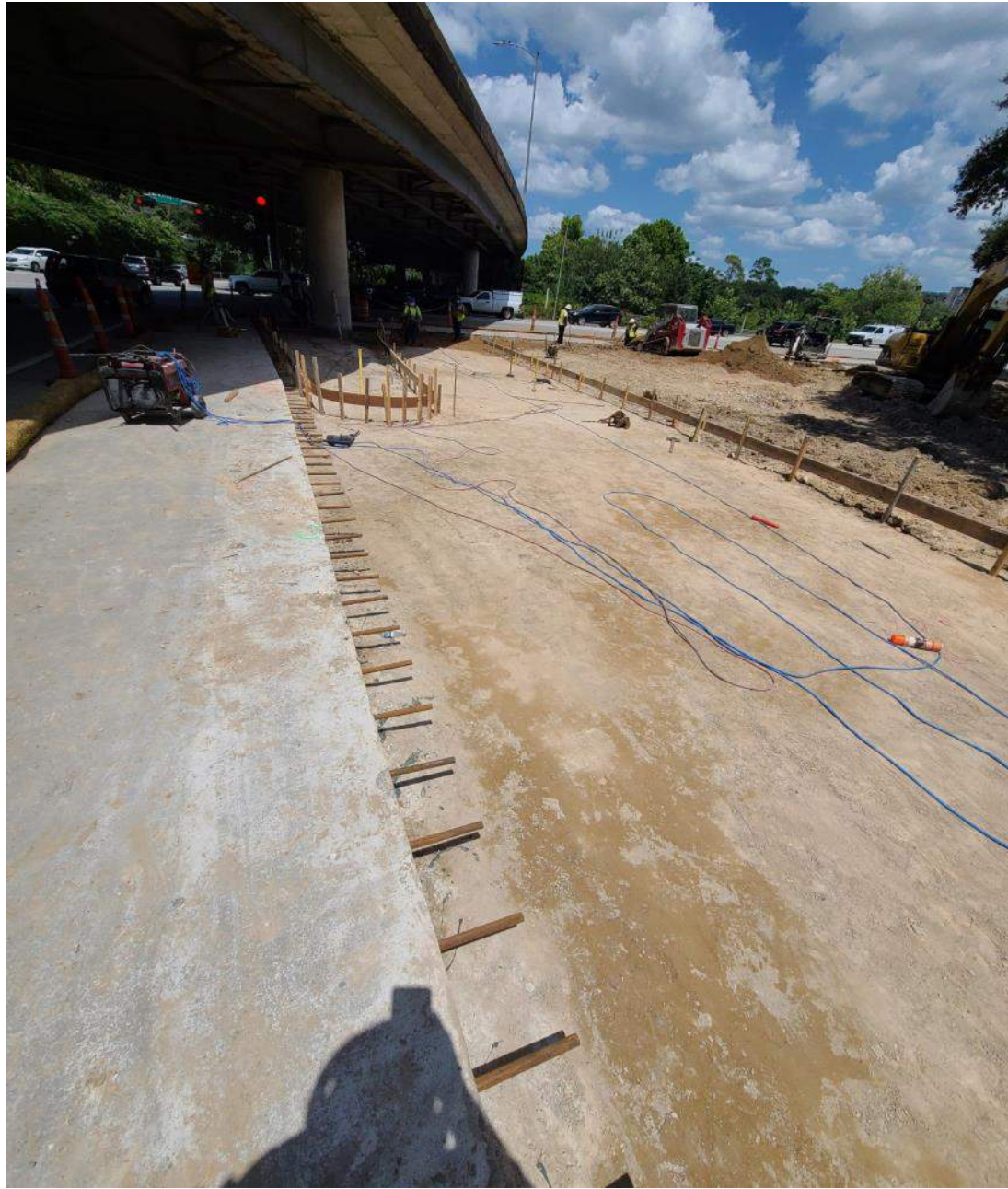
Formwork at Shepherd turn lane to Allen Pwky.
