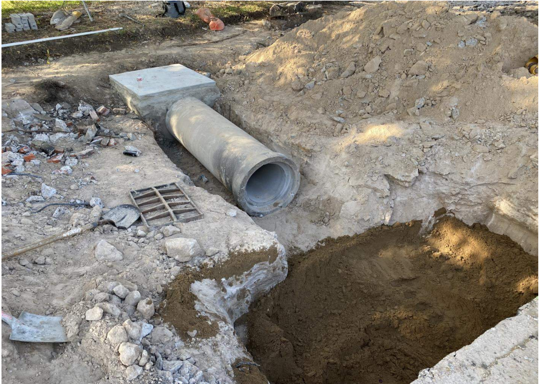
Jimerson installing new storm sewer Allen Pkwy.
